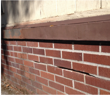
Cornelius ES: Missing mortar on exterior
