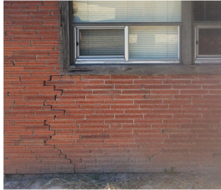
Harvey Clarke ES: Cracking in exterior brick
